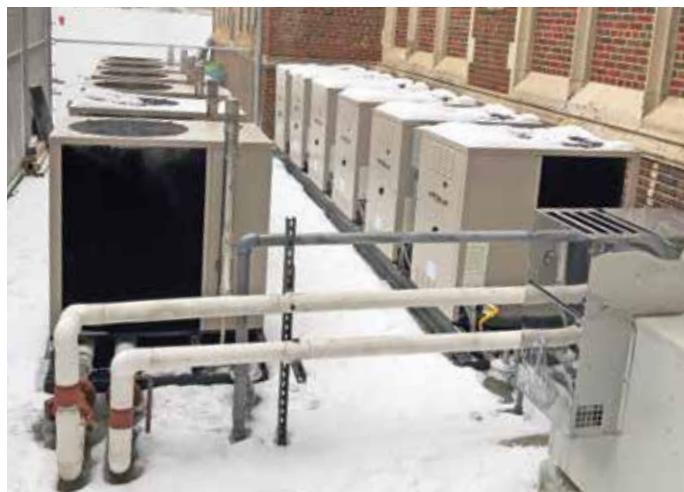
The Durfee Innovation Society used six Robur GAHP AR heat pumps and six Robur ACF60 ST chillers to provide heating and cooling for its 155,360-square-foot community center providing services for children, students and adults.
